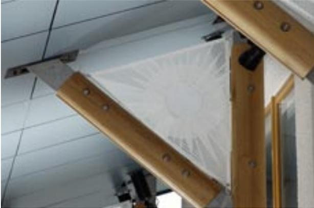
"I took the SAIL brief quite literally, and as a completely new departure for me, got involved with the new and exciting materials used by modern sail-makers. The materials finally selected were three different weights and constructions of clear, polyester laminates, stitched and glued to fit into the triangular sail-like shaped spaces at the top of the four entrance columns.
